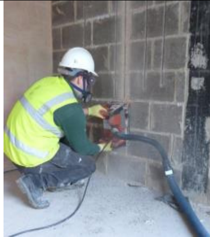
Good practice – Chasing concrete with on-tool extraction (HSE, GB)
