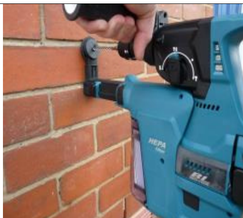
Good practice – Using a hand-held drill with integrated cassette (HSE, GB)
