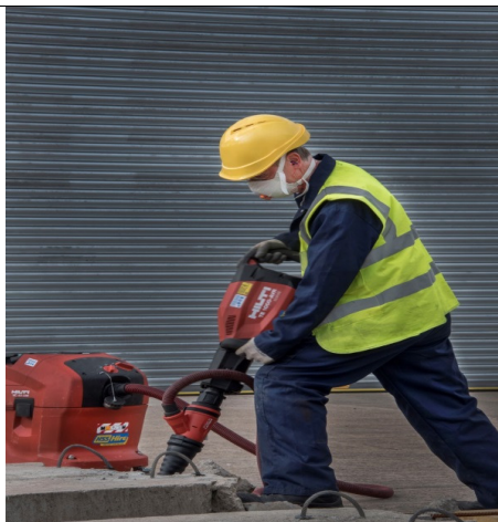
Good practice – Using a hand-held breaker with on-tool extraction (HSE, GB)
