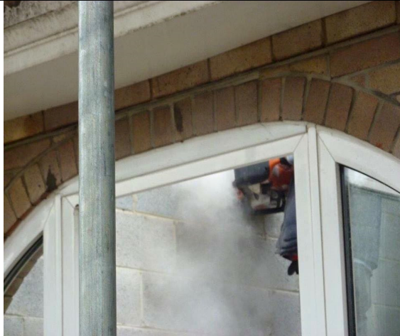
Poor Practice – Chasing concrete with no on-tool extraction or RPE (Safer Sites Website, GB)
