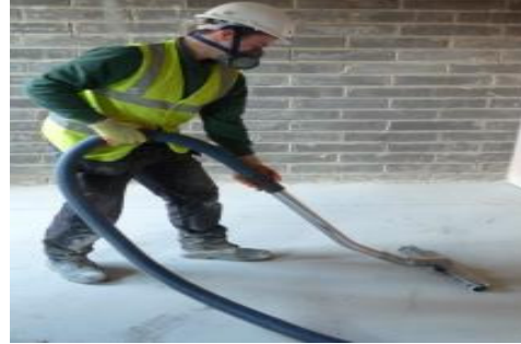
Good practice – Removal of dust using high-efficiency filter vacuum (HSE, GB)
