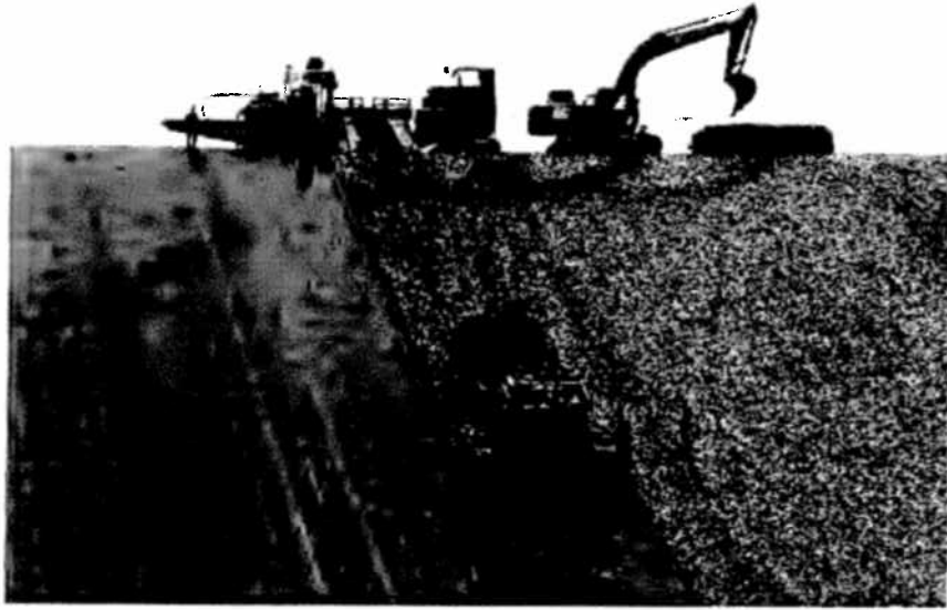
Paving of binder (pictured above) and barrier layer (below)
