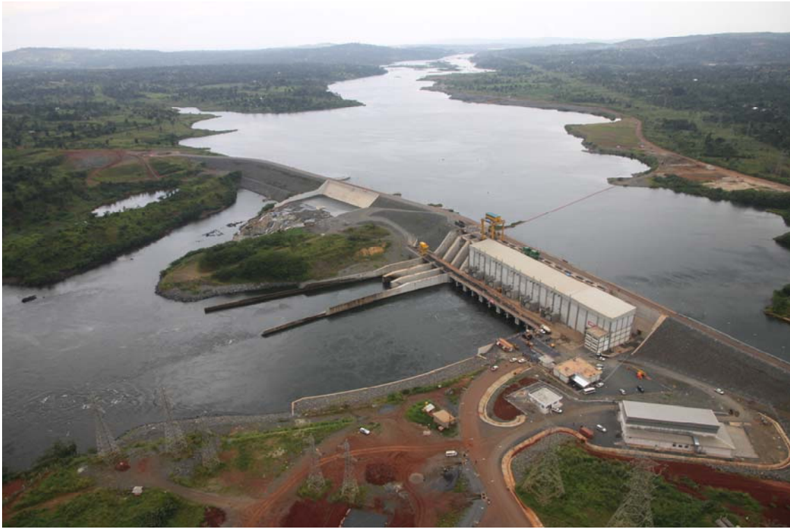
Salini - Bujagali Hydropower Project - Uganda
