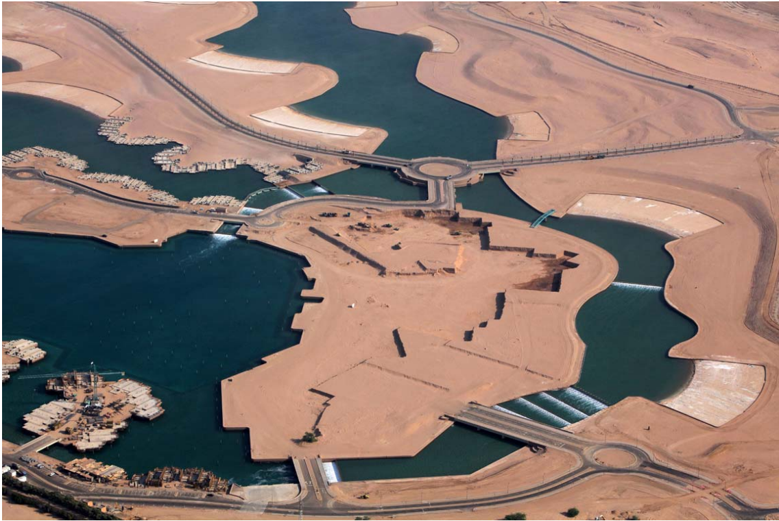
Condotte - Ayla Oasis Project – Jordan
